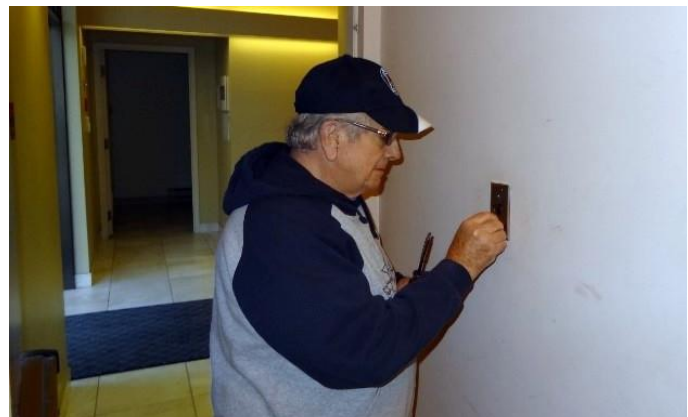
Sam is repairing the light switch leading to the basement
